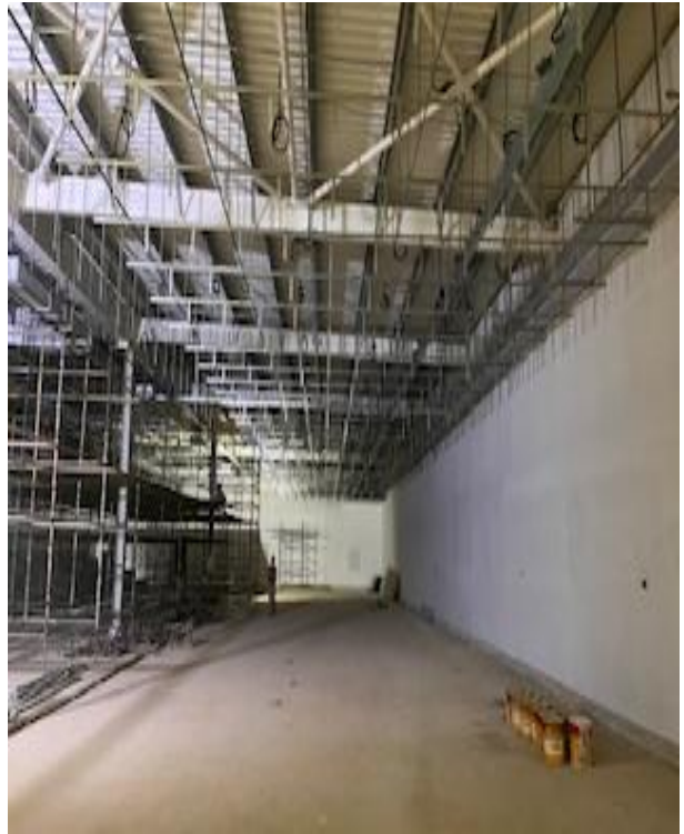
MOD SOUND ABSORBE CEILING FRAME WORK
