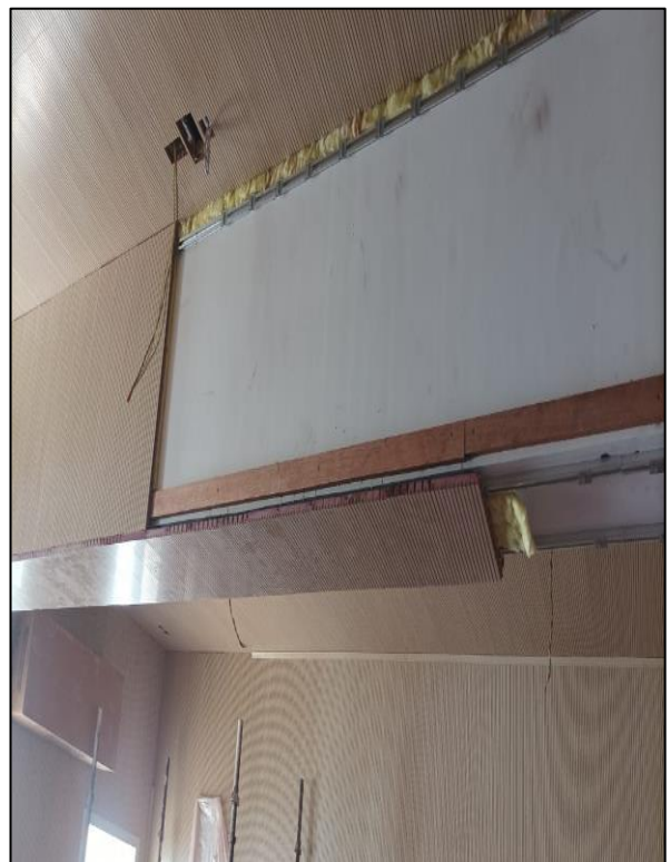
ACOUSTIC WALL PANELING WORK AT MOE
