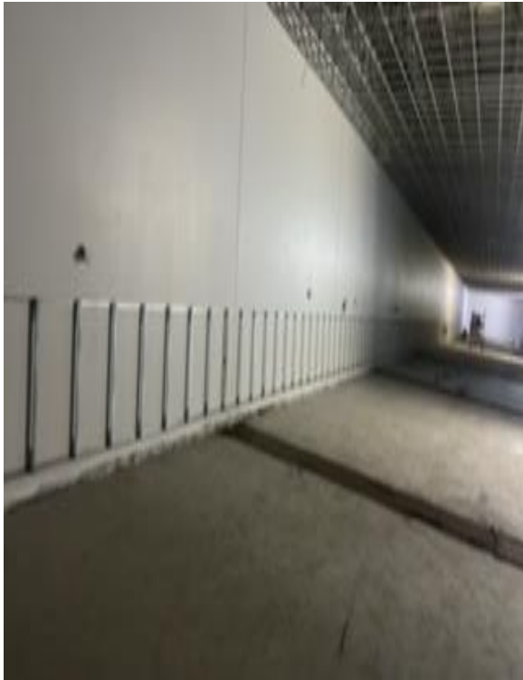
MOD WETHER BOARD CLADDING FRAME WORK
